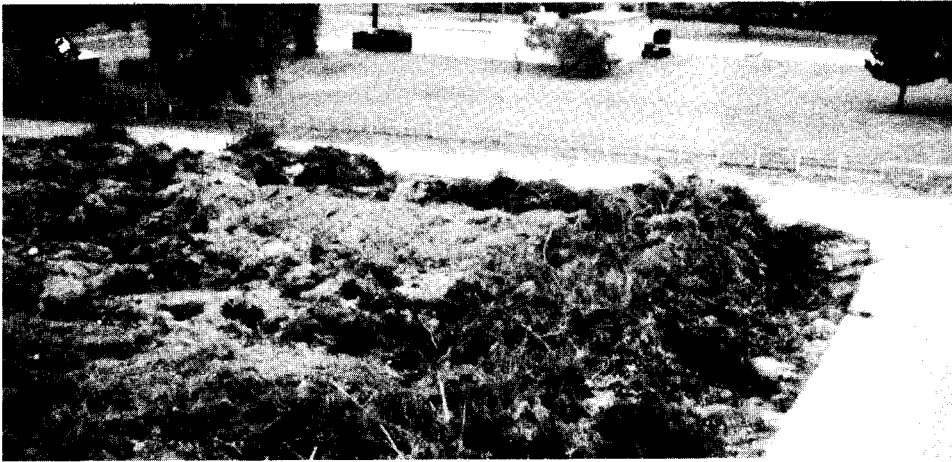
When the composting site is completed, it will be fully paved, fenced and landscaped with trees and flowers planted around the borders.
