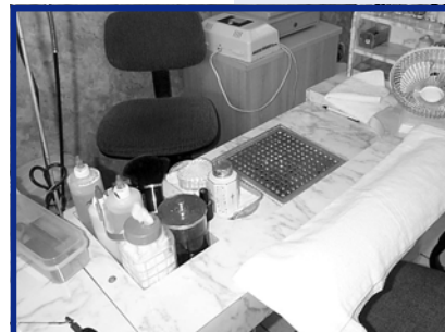
Exhaust vent embedded in nail care workstation
