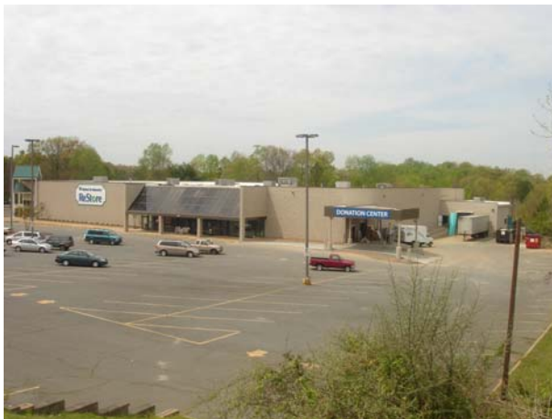
Habitat for Humanity Charlotte's new ReStore has more than 37,000 square feet of retail space for recovered building materials.
