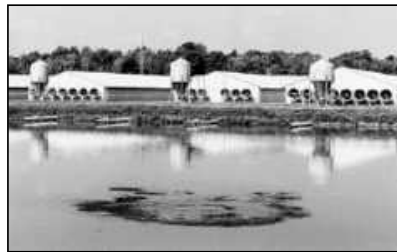
At Sarem Farms in Gates County, waste is funneled from pigs' quarters, in the background, to a lagoon where it bubbles up. When the solid waste is broken down into a liquid, it is processed and sprayed on fields at the farm.
