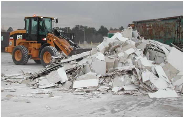
Drywall waste being consolidated at New Hanover County’s C&D recycling operation.
