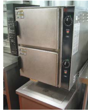
Figure 8. SC5 Hotel Main Kitchen and Boiler-based Steamer
