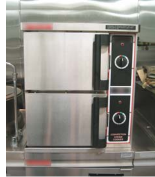
Figure 6. SC3 Corporate Cafeteria Kitchen and Boiler-based Steamer
