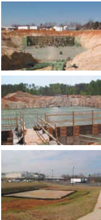
Below: Construction of the underground rainwater cistern at the school
